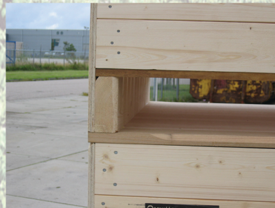
Closed pallet bottom which makes pallet ventilation possible
