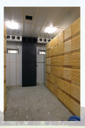
A room ventilation system creates an artificial airflow through the room. It is necessary to use standard open boxes. The air outlet is situated at the top of the system. The air is blown over the boxes to the other side of the room. As a result of the air suction from the bottom of the system the air circulation takes place through the boxes. An advantage of this system is a high storage capacity.
