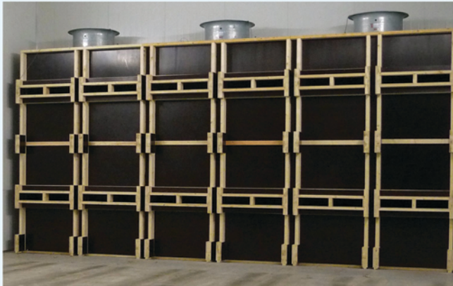
2-Layer ventilation wall
